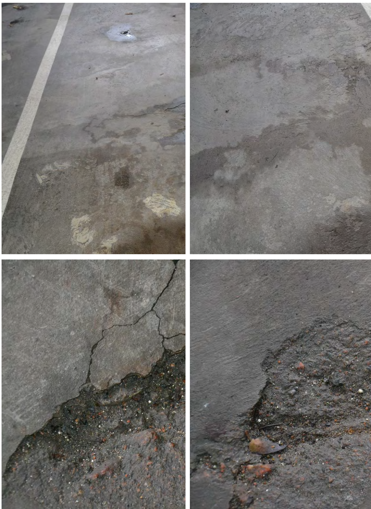
Figur 2.11 Skadad betong i garagage Kville
